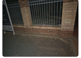
Item: Retaining walls
