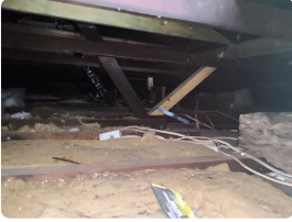
Item: Roof frame
