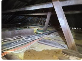
Item: Roof frame
