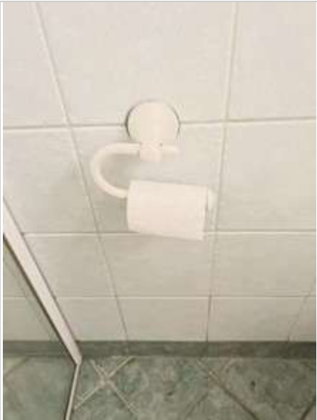
Bathroom 02/05/2023 1:55 PM Image 182 :Toilet Roll Holder
