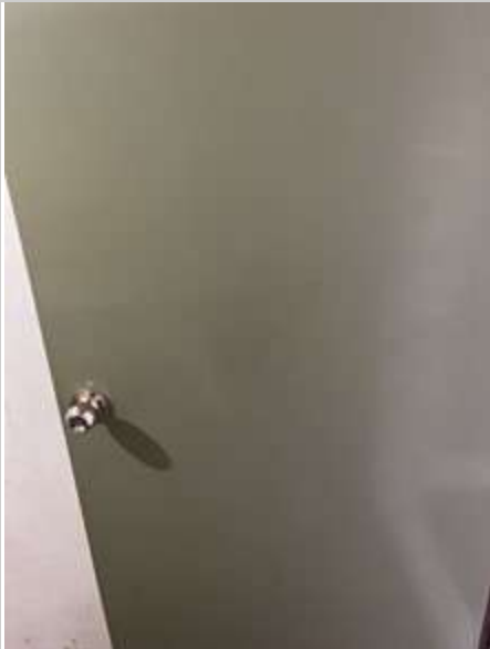
Storeroom 02/05/2023 3:07 PM Image 514 :Door/ Doorframe
