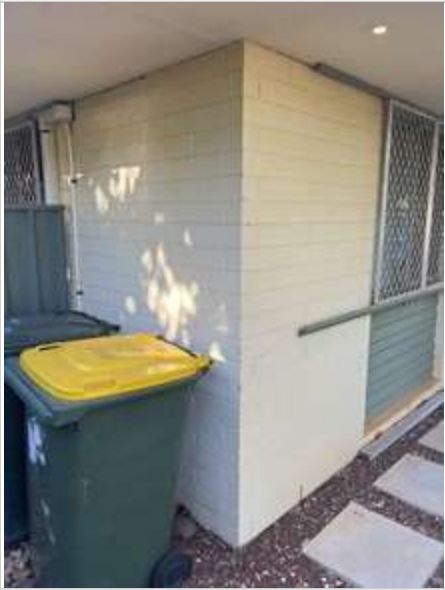
Exterior 02/05/2023 3:55 PM Image 420 :Walls And Fixtures
