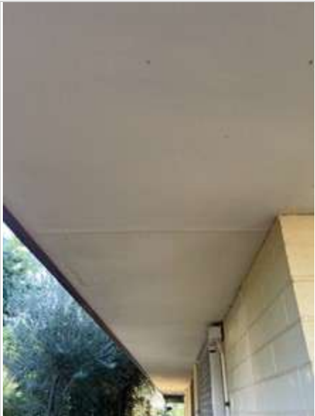
Exterior 02/05/2023 3:57 PM Image 498 :External Awnings
