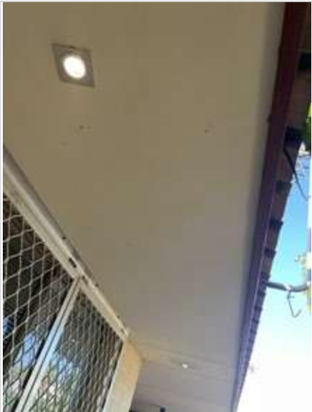
Exterior 02/05/2023 3:56 PM Image 486 :Front Porch/ Veran...
