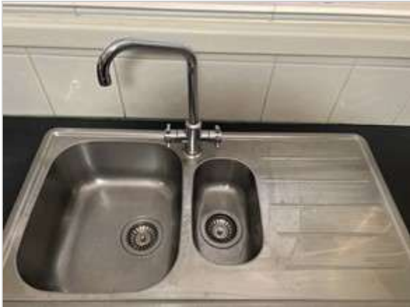
Kitchen 02/05/2023 2:54 PM Image 298 :Sink/ Taps
