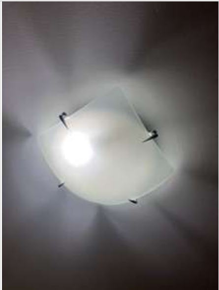
Dining Room 02/05/2023 3:48 PM Image 366 :Lights/ Fixtures
