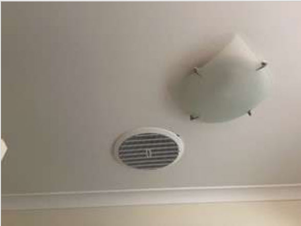
Bathroom 02/05/2023 1:59 PM Image 141 :Ceiling
