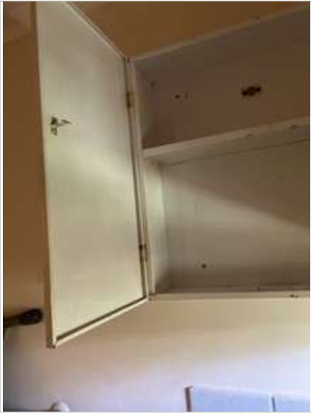
Laundry 02/05/2023 2:10 PM Image 380 :Cupboard
