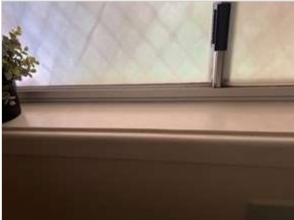
Bathroom 02/05/2023 1:56 PM Image 186 :Windows/ Screen...
