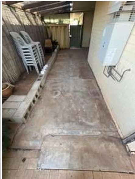
Exterior 02/05/2023 3:59 PM Image 491 :Front Porch/ Verand...
