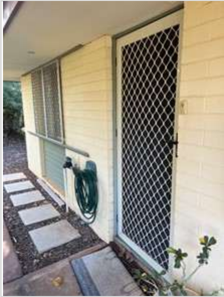
Exterior 02/05/2023 3:55 PM Image 419 :Walls And Fixtures
