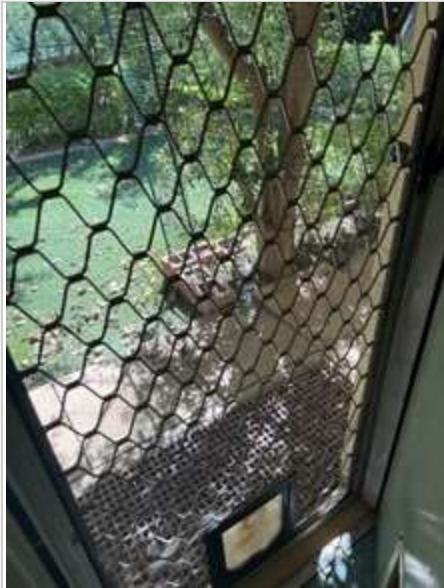
Laundry 02/05/2023 2:08 PM Image 403 :Door/ Doorframe
