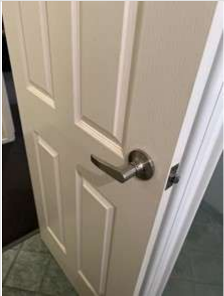
Bathroom 02/05/2023 2:00 PM Image 156 :Door/ Doorframe
