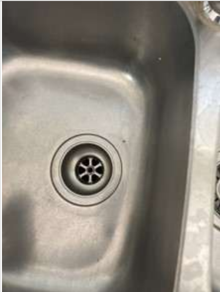
Kitchen 02/05/2023 2:54 PM Image 300 :Sink/ Taps
