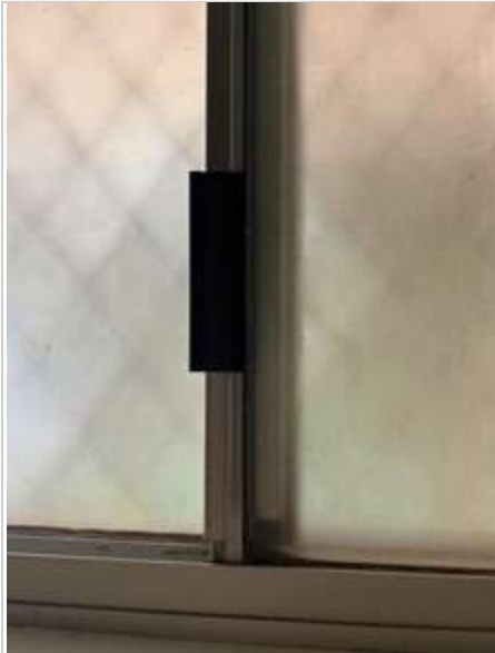
Bathroom 02/05/2023 1:56 PM Image 188 :Windows/ Screens/ ...
