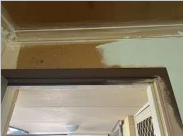
Storeroom 02/05/2023 3:08 PM Image 513 :Walls
