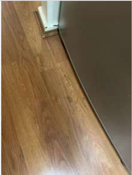
Kitchen 02/05/2023 2:50 PM Image 262 :Floor/ Tiles
