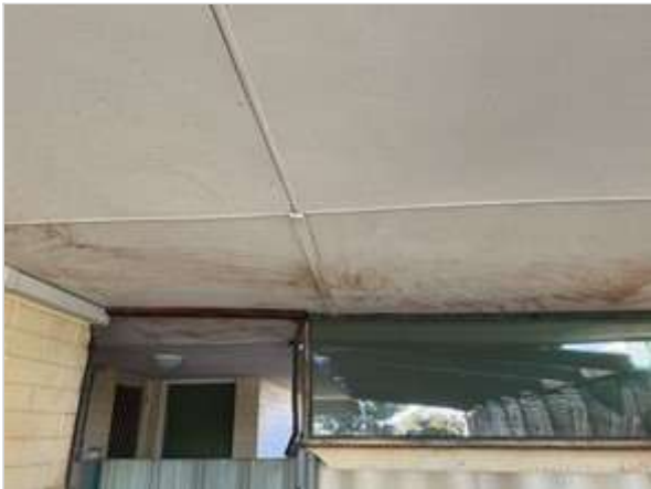
Exterior 02/05/2023 3:57 PM Image 496 :External Awnings
