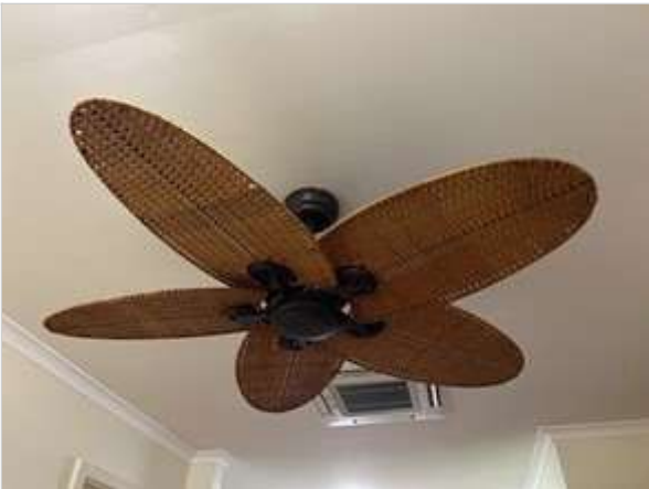
Dining Room 02/05/2023 3:48 PM Image 367 :Lights/ Fixtures
