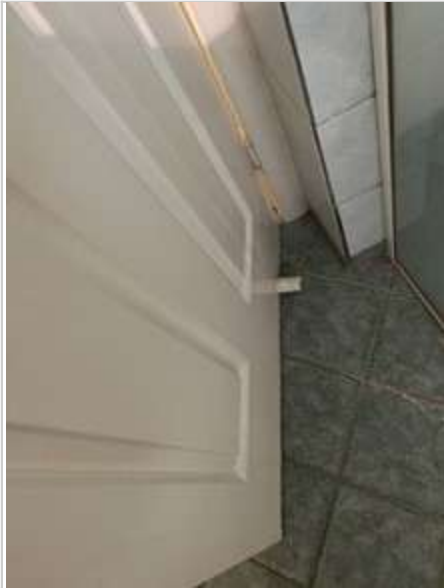
Bathroom 02/05/2023 2:00 PM Image 155 :Door/ Doorframe
