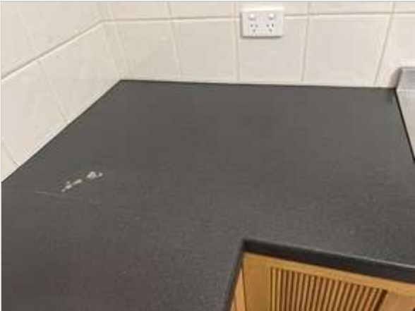
Kitchen 02/05/2023 2:53 PM Image 293 :Benchtops/ Tiling
