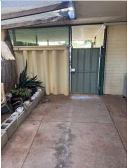
Exterior 02/05/2023 3:23 PM Image 432 :Gate/ Fence
