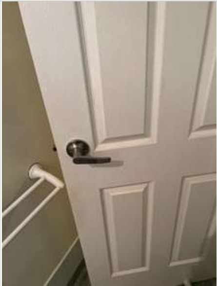
Bathroom 02/05/2023 2:00 PM Image 154 :Door/ Doorframe
