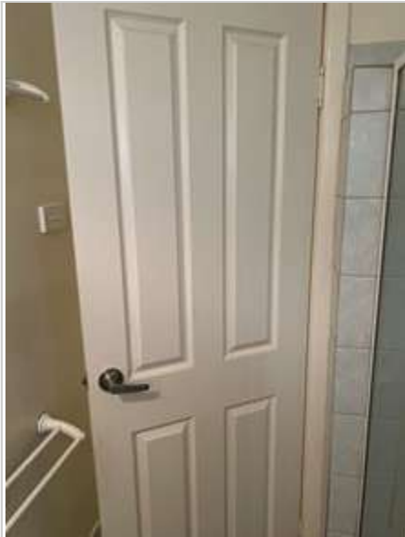
Bathroom 02/05/2023 1:59 PM Image 153 :Door/ Doorframe
