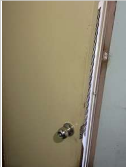
Storeroom 02/05/2023 3:07 PM Image 515 :Door/ Doorframe
