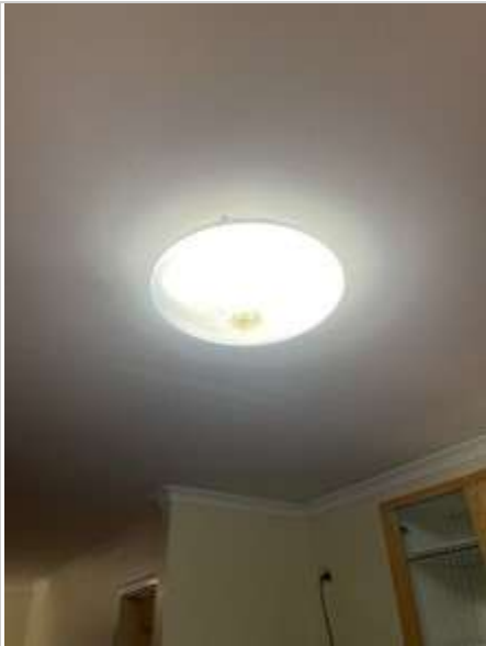
Kitchen 02/05/2023 3:01 PM Image 318 :Lights/ Fixtures
