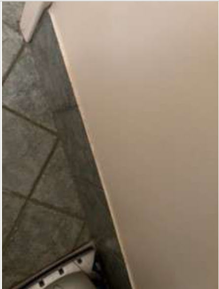
Laundry 02/05/2023 2:02 PM Image 390 :Walls/ Tiles
