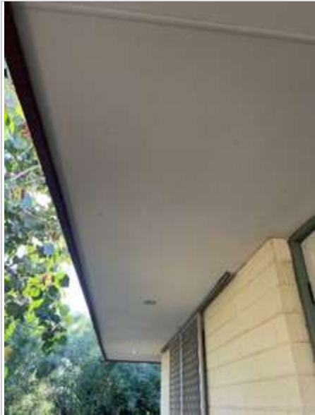
Exterior 02/05/2023 3:56 PM Image 487 :Front Porch/ Verand..
