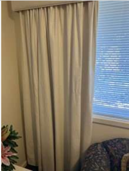
Lounge Room 02/05/2023 2:28 PM Image 132 :Blinds/ Curtains
