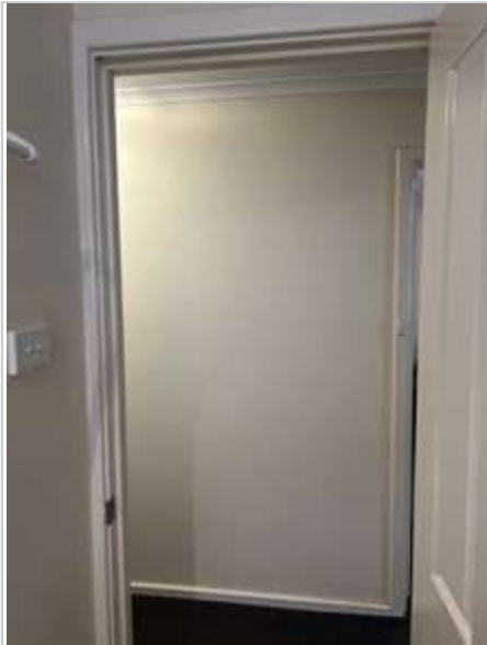
Bathroom 02/05/2023 2:00 PM Image 157 :Door/ Doorframe
