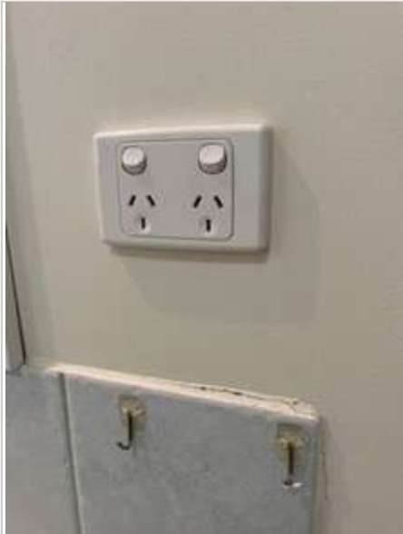
Bathroom 02/05/2023 1:47 PM Image 159 :Powerpoints/ Fixtures
