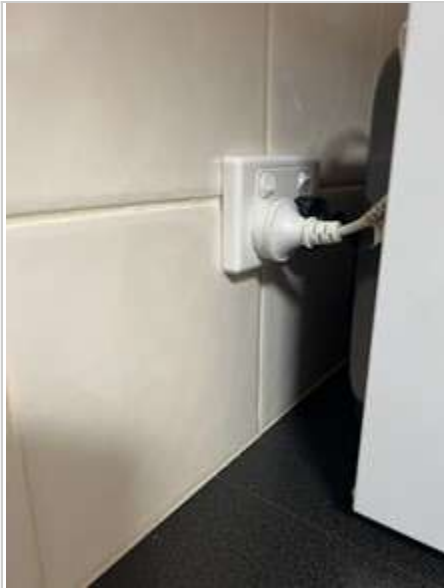
Kitchen 02/05/2023 2:51 PM Image 273 :Powerpoints/ Fixtures
