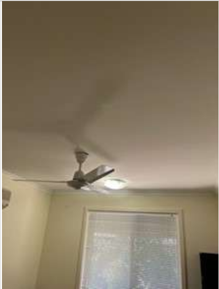
Bedroom 2 02/05/2023 2:17 PM Image 260 :Ceiling
