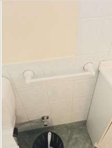
Bathroom 02/05/2023 1:55 PM Image 183 :Towel Rails
