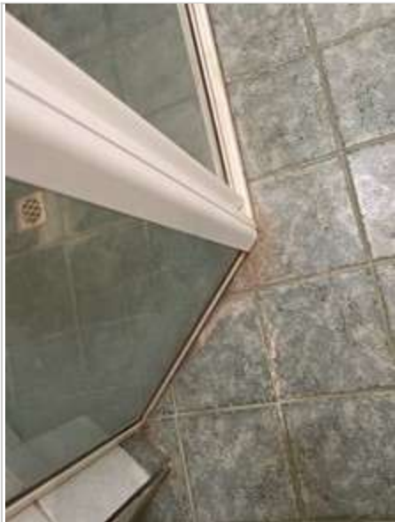
Bathroom 02/05/2023 1:45 PM Image 143 :Floor/ Tiles
