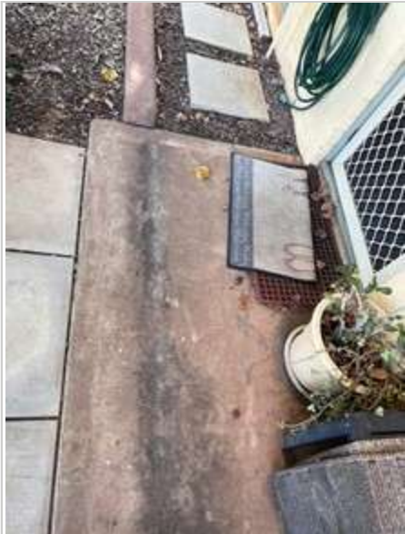
Exterior 02/05/2023 3:56 PM Image 485 :Front Porch/ Veran...
