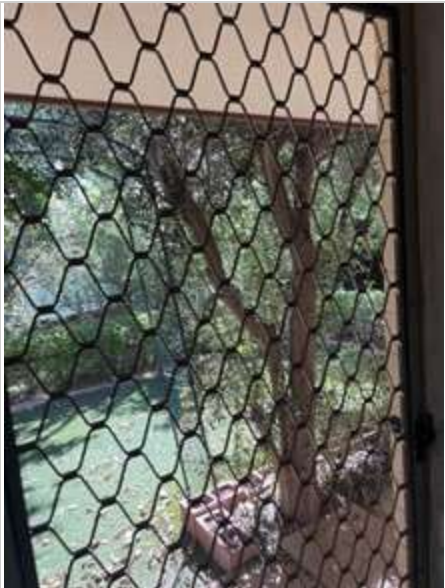
Laundry 02/05/2023 2:08 PM Image 402 :Door/ Doorframe
