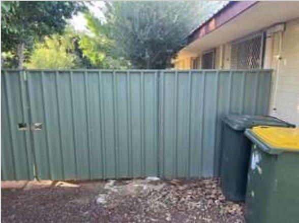
Exterior 02/05/2023 3:55 PM Image 437 :Gate/ Fence
