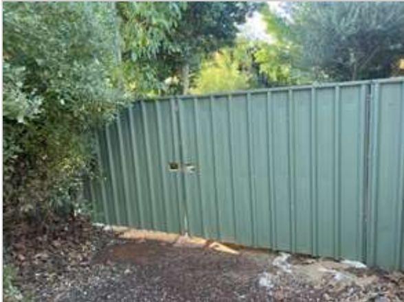
Exterior 02/05/2023 3:55 PM Image 438 :Gate/ Fence
