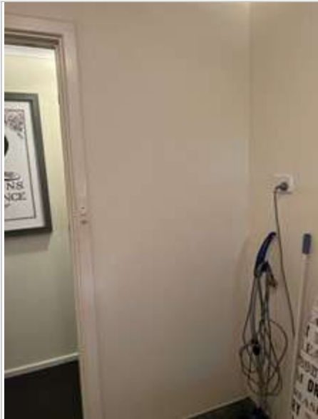
Laundry 02/05/2023 2:01 PM Image 385 :Walls/ Tiles
