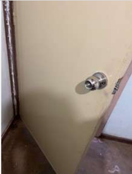
Storeroom 02/05/2023 3:07 PM Image 516 :Door/ Doorframe
