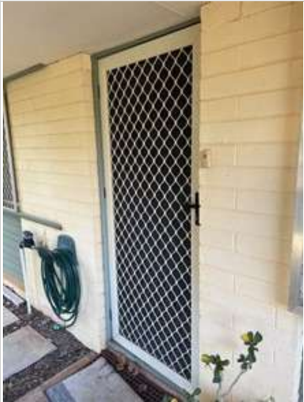
Exterior 02/05/2023 3:56 PM Image 484 :Front Porch/ Veran...
