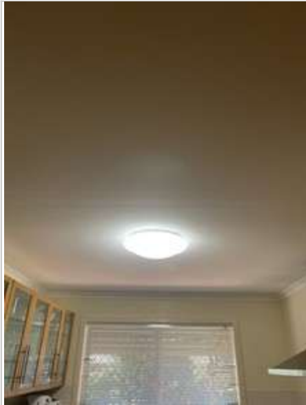
Kitchen 02/05/2023 3:02 PM Image 319 :Ceiling
