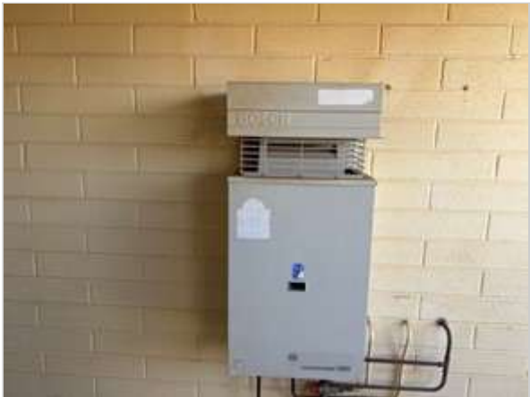
Exterior 02/05/2023 3:25 PM Image 412 :Walls And Fixtures
