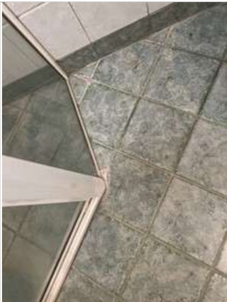
Bathroom 02/05/2023 1:45 PM Image 144 :Floor/ Tiles
