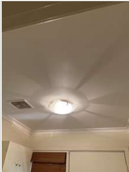
Laundry 02/05/2023 2:05 PM Image 411 :Ceiling
