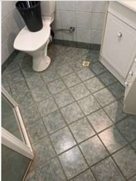
Bathroom 02/05/2023 1:45 PM Image 142 :Floor/ Tiles
