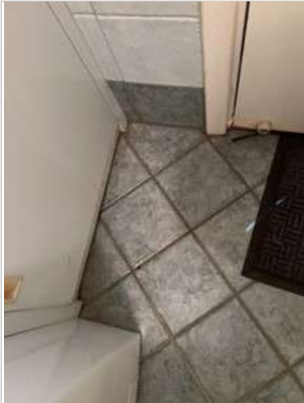
Laundry 02/05/2023 2:01 PM Image 383 :Floor/ Tiles
