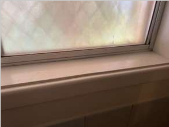
Bathroom 02/05/2023 1:56 PM Image 187 :Windows/ Screens/ ...
