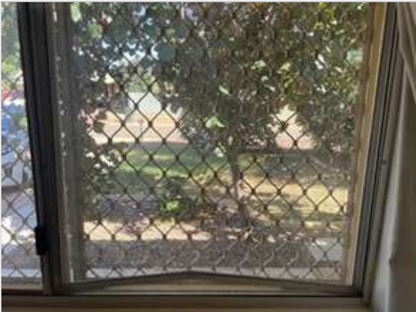
Lounge Room 02/05/2023 2:27 PM Image 129 :Windows/ Screens/ ...
