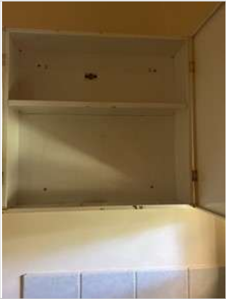
Laundry 02/05/2023 2:10 PM Image 378 :Cupboard
