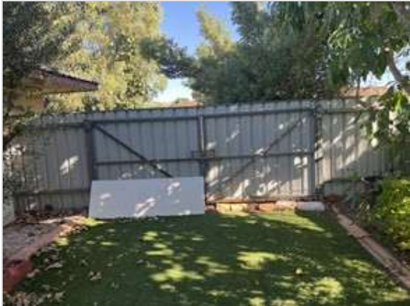
Exterior 02/05/2023 3:24 PM Image 436 :Gate/ Fence
