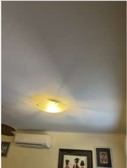
Lounge Room 02/05/2023 2:29 PM Image 138 :Ceiling
