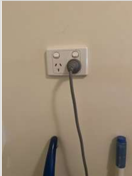
Laundry 02/05/2023 2:04 PM Image 405 :Powerpoints/ Fixtu...
