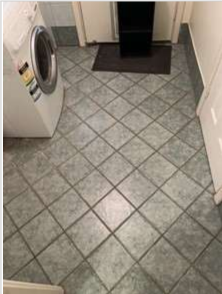
Laundry 02/05/2023 2:01 PM Image 381 :Floor/ Tiles
