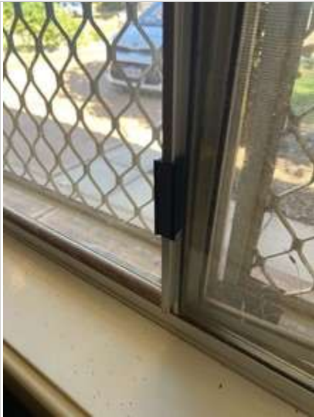
Lounge Room 02/05/2023 2:27 PM Image 130 :Windows/ Screens/ ...
