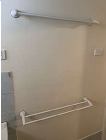
Bathroom 02/05/2023 1:55 PM Image 184 :Towel Rails
