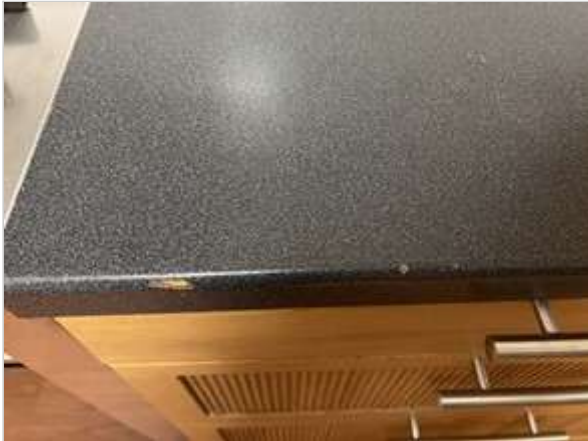
Kitchen 02/05/2023 2:53 PM Image 296 :Benchtops/ Tiling
