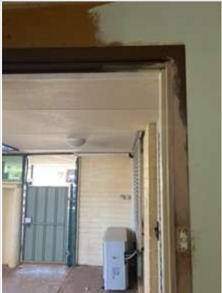
Storeroom 02/05/2023 3:08 PM Image 518 :Door/ Doorframe
