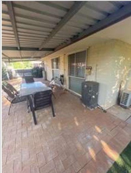
Exterior 02/05/2023 3:59 PM Image 489 :Front Porch/ Veran...
