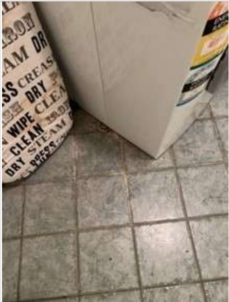
Laundry 02/05/2023 2:01 PM Image 382 :Floor/ Tiles
