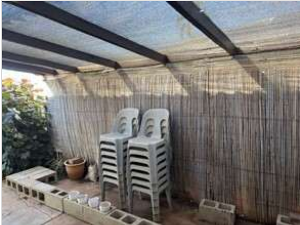
Exterior 02/05/2023 4:00 PM Image 440 :Gate/ Fence
