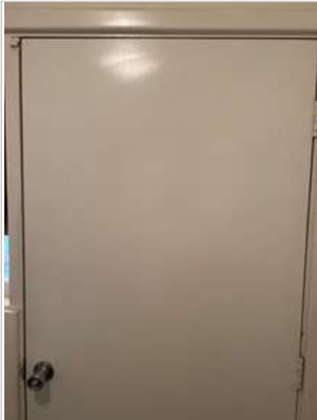
Laundry 02/05/2023 2:08 PM Image 401 :Door/ Doorframe
