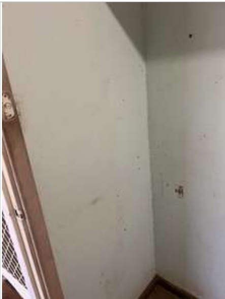
Storeroom 02/05/2023 3:05 PM Image 508 :Walls
