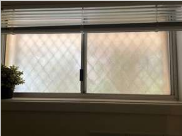
Bathroom 02/05/2023 1:56 PM Image 185 :Windows/ Screens/ ...
