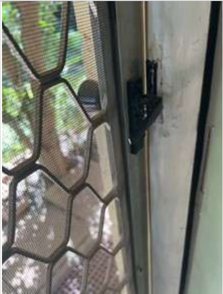
Laundry 02/05/2023 2:08 PM Image 404 :Door/ Doorframe
