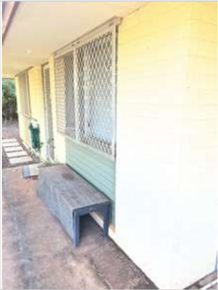
Exterior 02/05/2023 3:55 PM Image 418 :Walls And Fixtures
