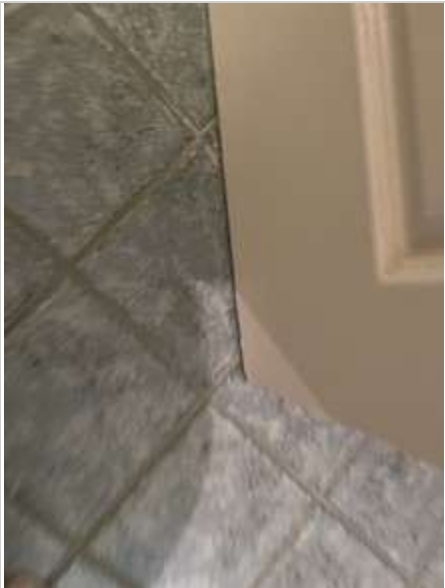
Bathroom 02/05/2023 2:00 PM Image 158 :Door/ Doorframe
