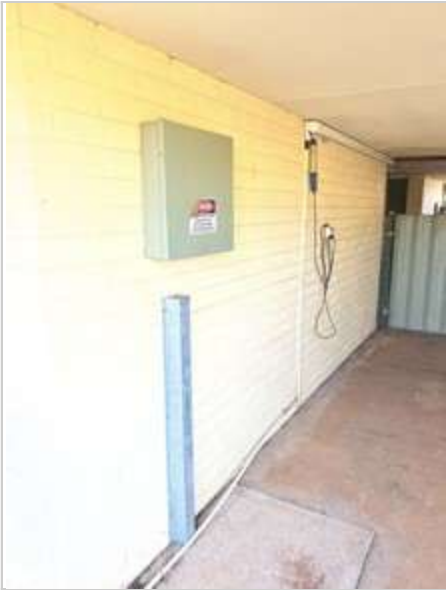
Exterior 02/05/2023 3:54 PM Image 417 :Walls And Fixtures
