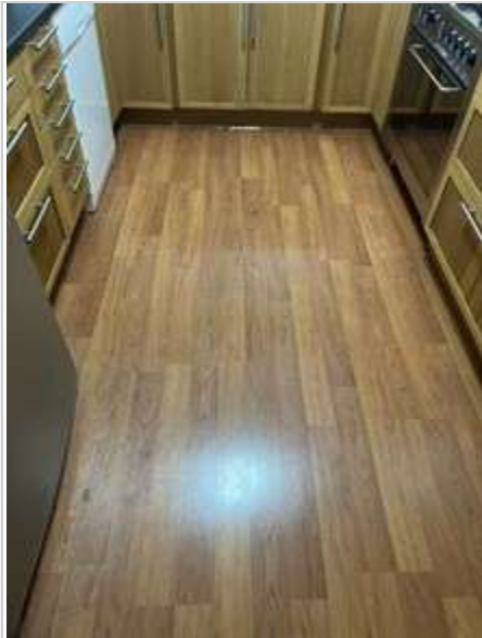
Kitchen 02/05/2023 2:50 PM Image 261 :Floor/ Tiles
