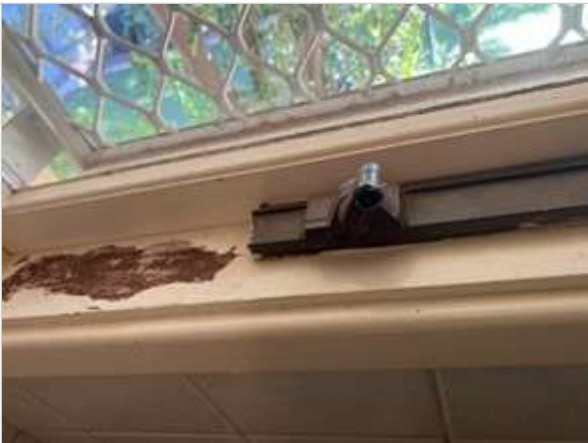
Laundry 02/05/2023 2:04 PM Image 407 :Windows/ Screens/ ...
