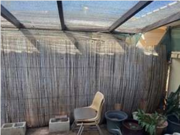
Exterior 02/05/2023 4:00 PM Image 439 :Gate/ Fence
