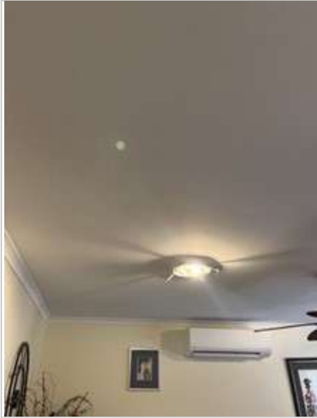
Lounge Room 02/05/2023 2:29 PM Image 139 :Ceiling
