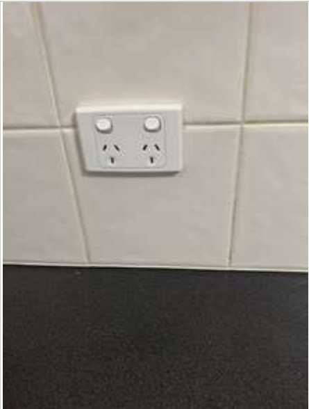
Kitchen 02/05/2023 2:51 PM Image 274 :Powerpoints/ Fixtures
