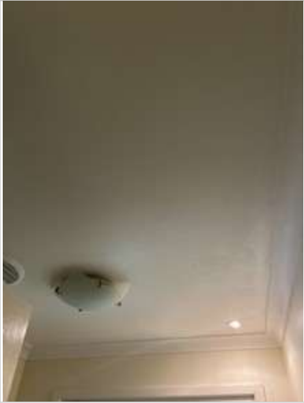
Bathroom 02/05/2023 1:59 PM Image 140 :Ceiling
