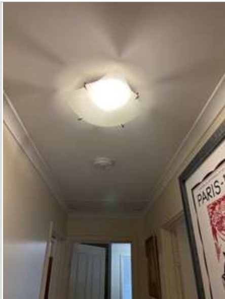
Hallway 02/05/2023 2:40 PM Image 95 :Lights
