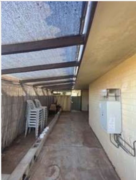
Exterior 02/05/2023 3:59 PM Image 492 :Front Porch/ Verand...
