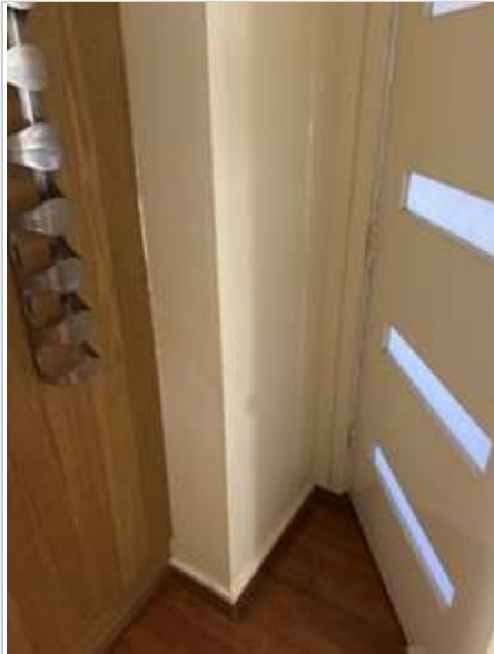
Dining Room 02/05/2023 3:42 PM Image 335 :Walls
