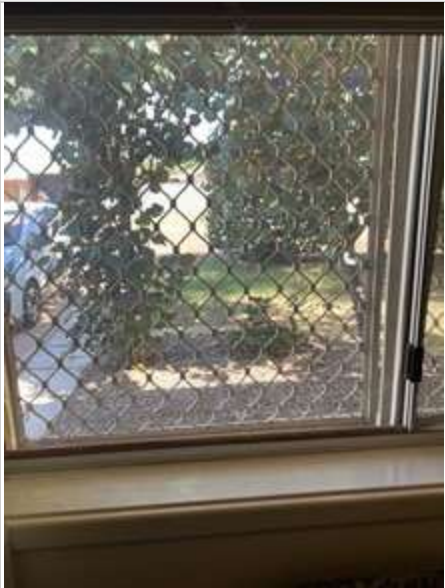
Lounge Room 02/05/2023 2:27 PM Image 128 :Windows/ Screens/ ...
