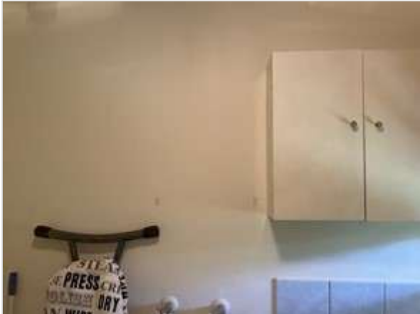
Laundry 02/05/2023 2:01 PM Image 384 :Walls/ Tiles
