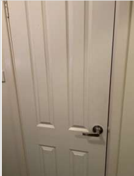
Laundry 02/05/2023 2:06 PM Image 372 :Cupboard
