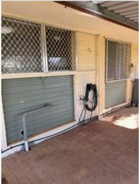
Exterior 02/05/2023 3:25 PM Image 414 :Walls And Fixtures
