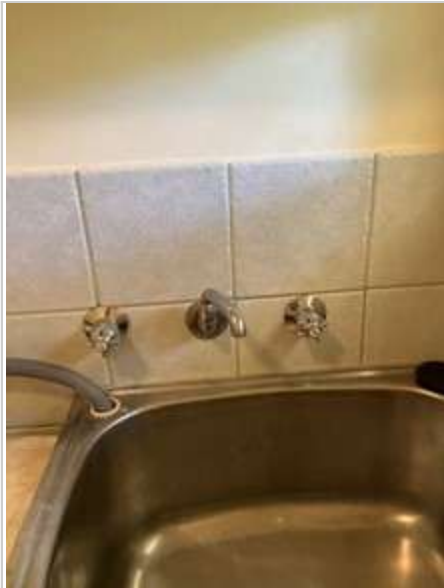
Laundry 02/05/2023 2:02 PM Image 393 :Walls/ Tiles
