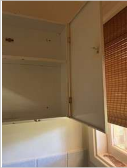
Laundry 02/05/2023 2:10 PM Image 379 :Cupboard
