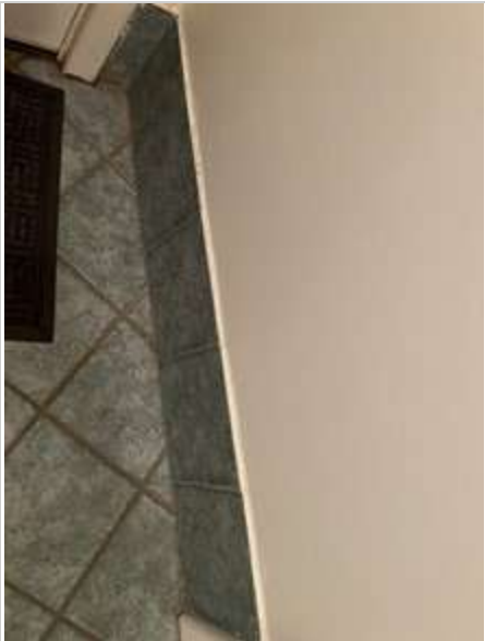
Laundry 02/05/2023 2:02 PM Image 394 :Walls/ Tiles
