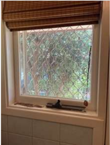
Laundry 02/05/2023 2:04 PM Image 406 :Windows/ Screens/ ...
