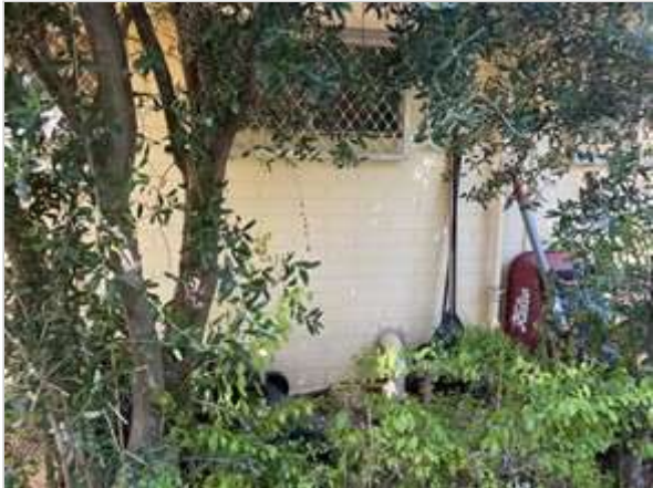
Exterior 02/05/2023 3:26 PM Image 416 :Walls And Fixtures
