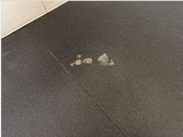
Kitchen 02/05/2023 2:53 PM Image 294 :Benchtops/ Tiling
