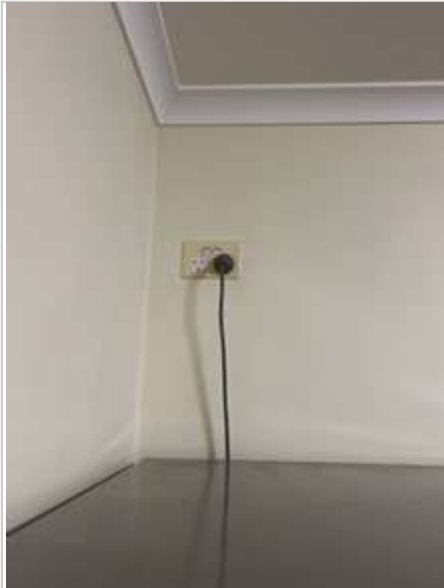
Kitchen 02/05/2023 3:02 PM Image 275 :Powerpoints/ Fixtures
