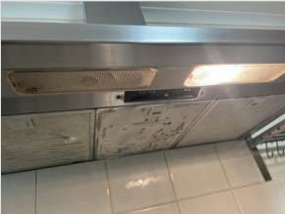
Kitchen 02/05/2023 3:00 PM Image 313 :Exhaust Fan/ Rangeh..
