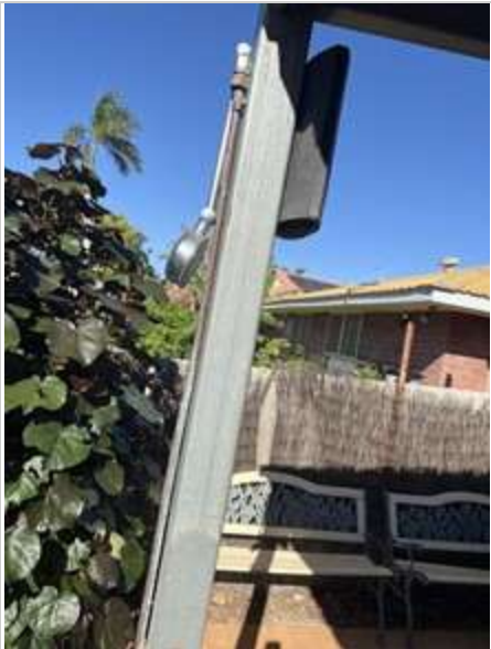
Exterior 02/05/2023 3:19 PM Image 482 :Front Porch/ Verand..
