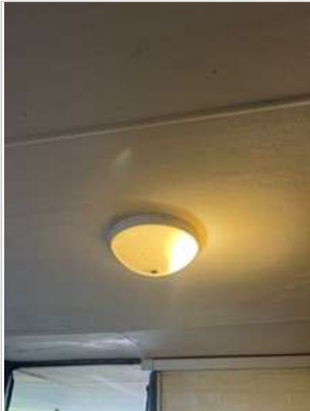
Exterior 02/05/2023 4:00 PM Image 493 :Front Porch/ Veran...
