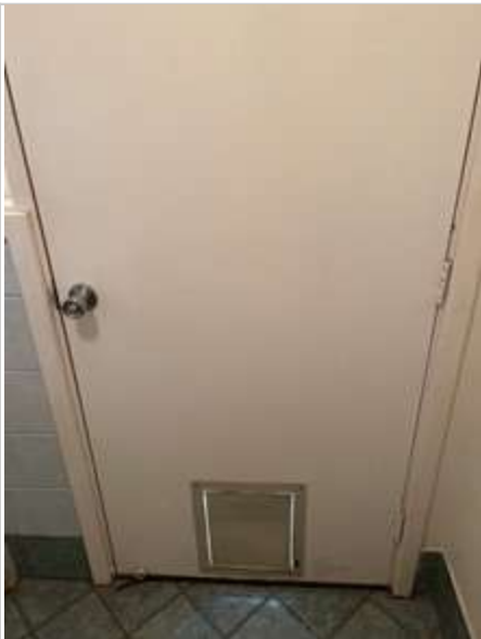
Laundry 02/05/2023 2:08 PM Image 400 :Door/ Doorframe
