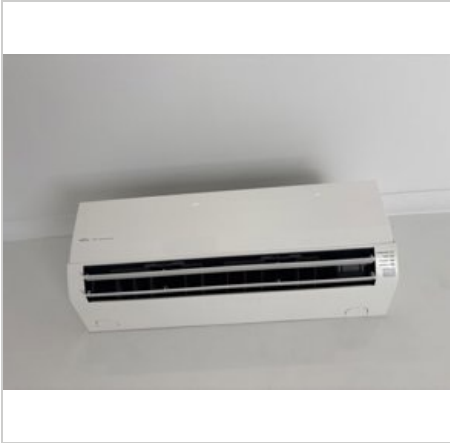
Lounge Room 17/03/2025 3:16 PM Image 93 :Powerpoints/ Fixtures
