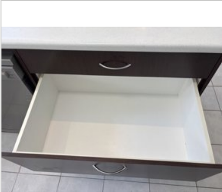
Kitchen 17/03/2025 2:52 PM Image 327 :Cupboards
