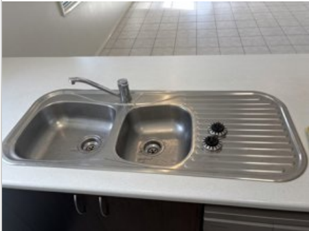
Kitchen 17/03/2025 2:57 PM Image 367 :Sink/ Taps
