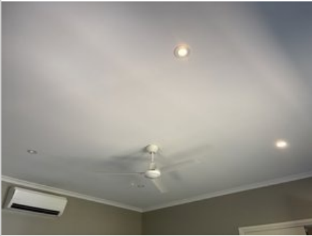
Family room 17/03/2025 2:16 PM Image 470 :Lights/ Fixtures
