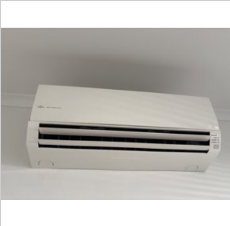
Bedroom 2 17/03/2025 3:40 PM Image 586 :Powerpoints/ Fixtures
