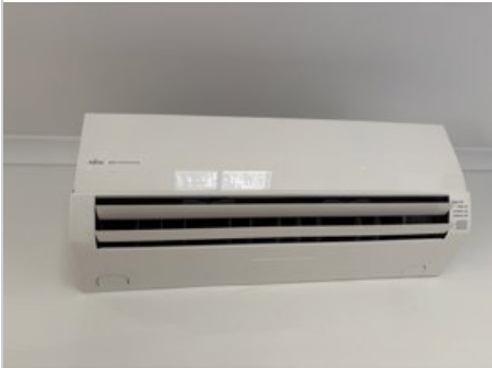
Bedroom 17/03/2025 2:25 PM Image 171 :Powerpoints/ Fixtures
