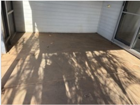
Exterior 17/03/2025 4:15 PM Image 966 :External Awnings
