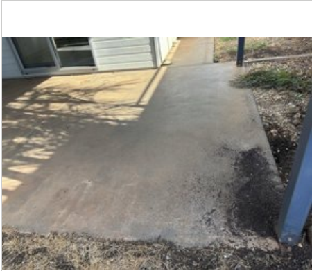
Exterior 17/03/2025 4:15 PM Image 965 :External Awnings
