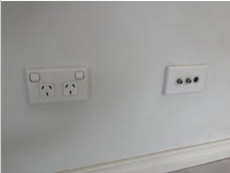
Lounge Room 17/03/2025 3:16 PM Image 88 :Powerpoints/ Fixtures
