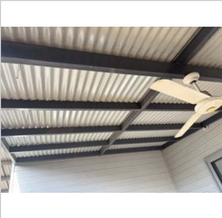
Exterior 17/03/2025 4:15 PM Image 969 :External Awnings
