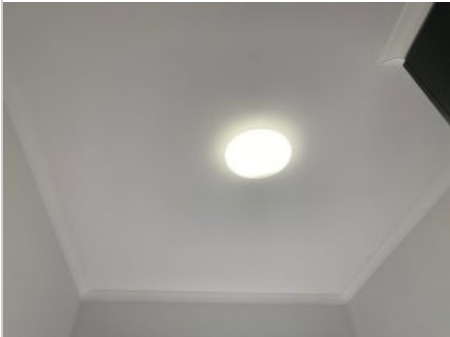
Laundry 17/03/2025 4:31 PM Image 911 :Ceiling
