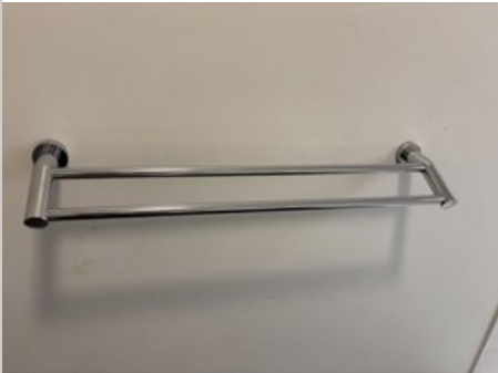
Bathroom 17/03/2025 4:11 PM Image 820 :Towel Rails
