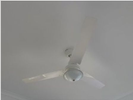
Bedroom 4 17/03/2025 4:00 PM Image 727 :Powerpoints/ Fixtures
