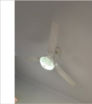
Bedroom 3 17/03/2025 3:51 PM Image 663 :Powerpoints/ Fixtures
