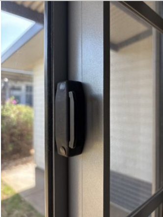
Bedroom 17/03/2025 2:26 PM Image 173 :Windows/ Screens/ Window Saf...
