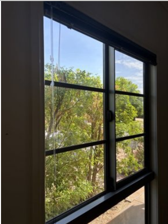
Bedroom 17/03/2025 2:26 PM Image 175 :Windows/ Screens/ Window Saf...
