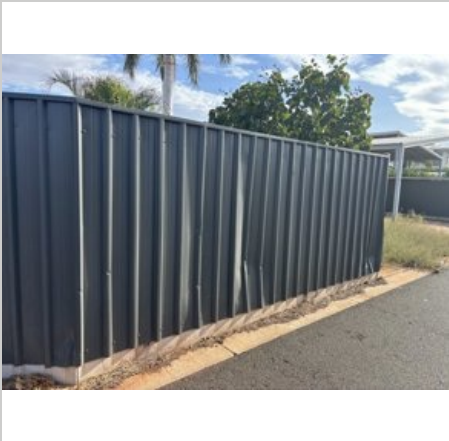
Exterior 17/03/2025 4:19 PM Image 922 :Gate/ Fence
