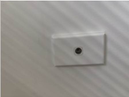
Bedroom 4 17/03/2025 4:00 PM Image 728 :Powerpoints/ Fixtures
