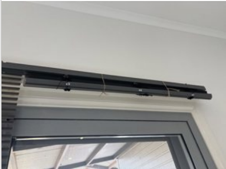
Lounge Room 17/03/2025 3:18 PM Image 115 :Blinds/ Curtains
