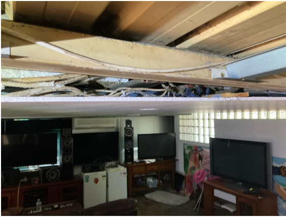
Exposed wiring junctions observed in the roof void above the patio area.
