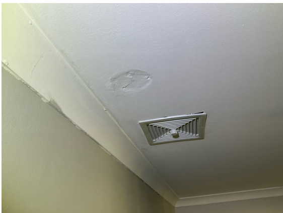
Bed 5 - Minor damage noted to ceiling lining at isolated areas throughout the home. Recommend maintenance/repair.
