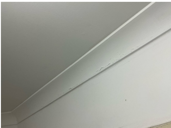
Ensuite - Flakey paint noted to cornice. Recommend maintenance/repair and paint.
