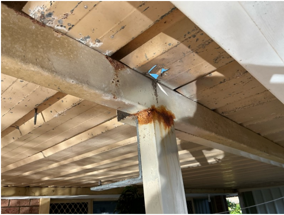
Surface rust noted to patio structure to some areas throughout the home. Recommend to treat rust and paint with protective coating.
