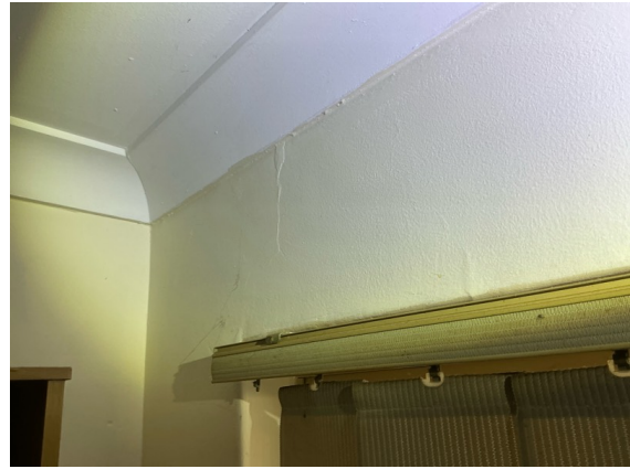
Laundry - Typical appearance cracking noted to wall linings at some isolated areas throughout the home. Recommend maintenance/repairs and to monitor over time.
