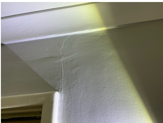
Bathroom - Typical appearance cracking noted to wall linings at some isolated areas throughout the home. Recommend maintenance/repairs and to monitor over time.
