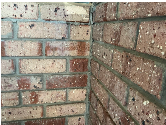
Carport - Appearance wall cracking to some external brickwork. Recommend maintenance / Repair and monitor over time.
