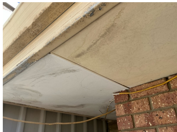
East Elevation - Joining strip disengaged from eaves lining. Recommend maintenance/repair.
