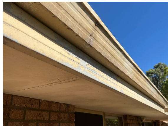
Rust damaged fascia, gutters and down pipes were observed to various areas around the home. Recommend repairs/replacement.
