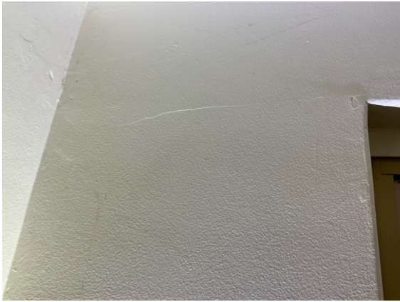
Meals - Typical appearance cracking noted to wall linings at some isolated areas throughout the home. Recommend maintenance/repairs and to monitor over time.
