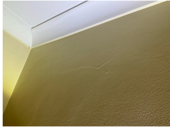
Bed 1 - Typical appearance cracking noted to wall linings at some isolated areas throughout the home. Recommend maintenance/repairs and to monitor over time.
