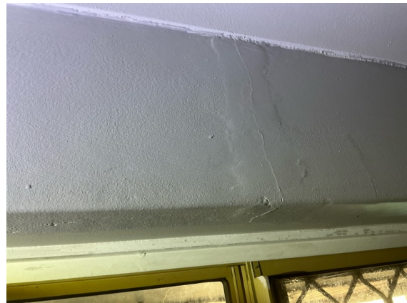
Bed 5 - Appearance cracking and patching noted to wall linings at some isolated areas throughout the home. Recommend maintenance/repairs and to monitor over time.
