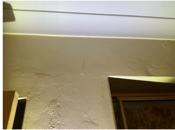
Bed 3 - Appearance cracking and patching noted to wall linings at some isolated areas throughout the home. Recommend maintenance/repairs and to monitor over time.
