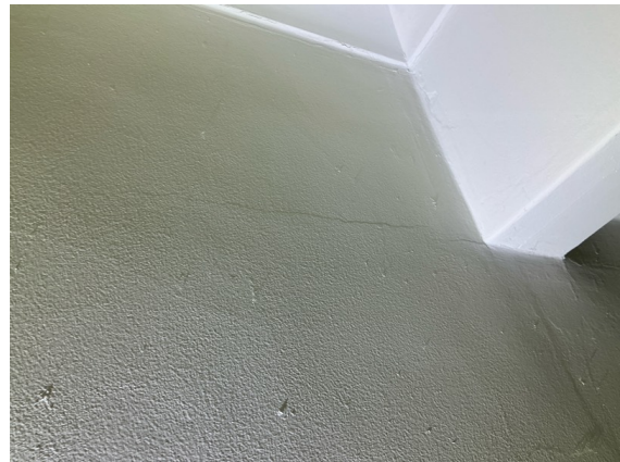
Ensuite - Typical appearance cracking noted to wall linings at some isolated areas throughout the home. Recommend maintenance/repairs and to monitor over time.
