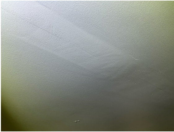
Appearance cracking noted to the ceiling lining at some isolated areas. Recommend maintenance/repairs.
