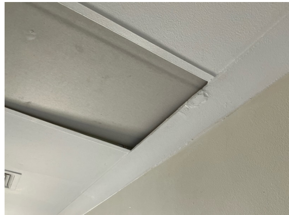
Hallway - Minor damage noted to ceiling cornice. Recommend maintenance/repair.
