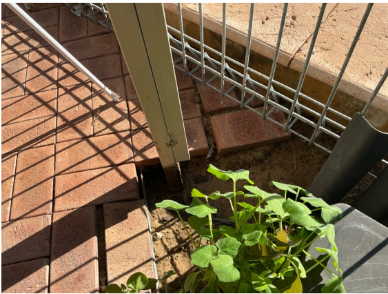
South Elevation - Some down pipes discharge next to the home. Recommend connecting all down pipes to stormwater system.
