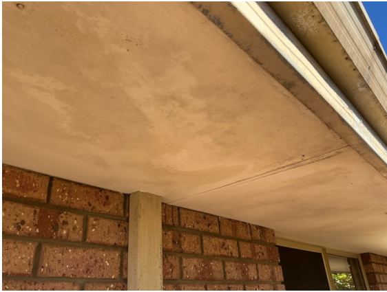
North Elevation - Evidence of moisture ingress to the exterior eaves lining in some areas. Eaves can be highly susceptible to moisture, often as a result of blocked and/or leaking gutters or down pipe connections. Recommend roof cover inspection, repairs and/or routine clearing of overflow provisions to gutters and down pipes as required.
