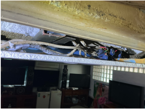
Exposed wiring junctions observed in the roof void above the patio area. Recommend having an Electrician install junction box's at all connections to make safe.
