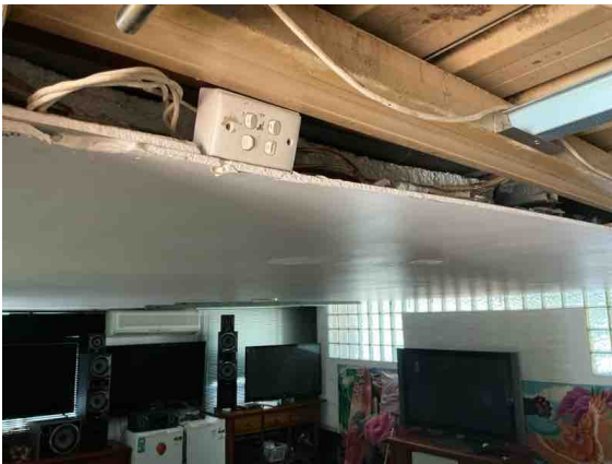
Opening to the roof void of the patio on the south side and exposed wiring is visible.
