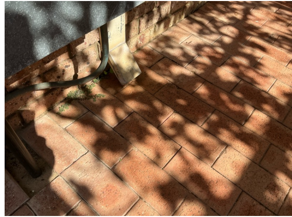
North Elevation - Some down pipes discharge next to the home. Recommend connecting all down pipes to stormwater system.
