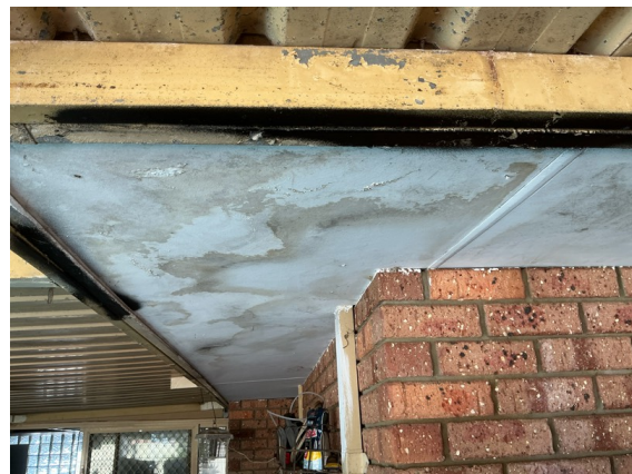
South Elevation - Evidence of moisture ingress to the exterior eaves lining in some areas. Eaves can be highly susceptible to moisture, often as a result of blocked and/or leaking gutters or down pipe connections. Recommend roof cover inspection, repairs and/or routine clearing of overflow provisions to gutters and down pipes as required.
