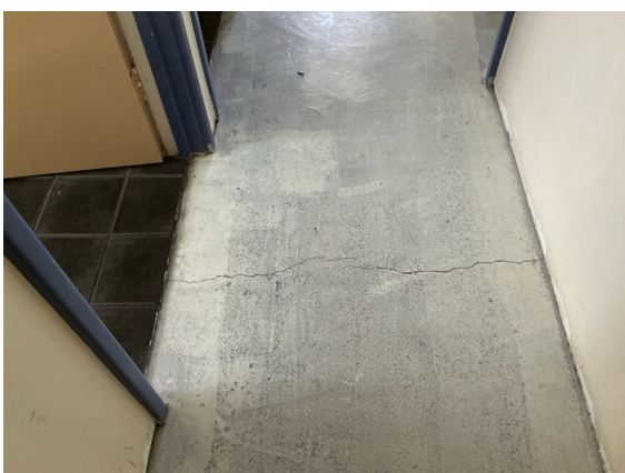
Hallway - Minor and typical appearance cracking was observed to various concrete floor finishes at some isolated areas throughout the home.
