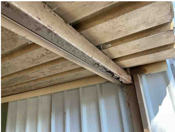
Significant rust noted to External patio structure to some areas. Recommend repairs or replacement.
