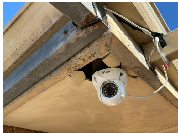
North Elevation - Minor damage noted to eaves lining at isolated areas throughout the home. Recommend maintenance/repair.
