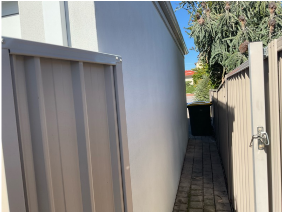
West elevation garage wall
