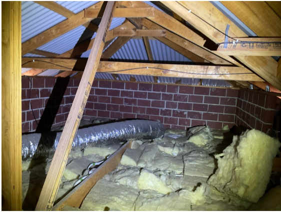
South elevation roof void
