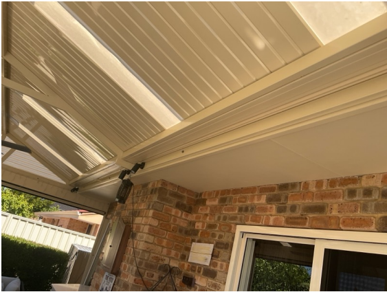
Patio connections to the main residence are adequate and performing on day of inspection
