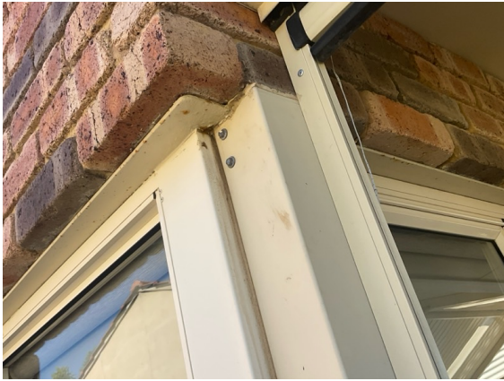
Evidence of surface rust noted to the west elevation external brick opening lintels. This is common when maintenance painting is not carried out. Recommend treat and paint
