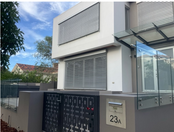
Eastern elevation. Exterior walls and some elements have been recently painted.
