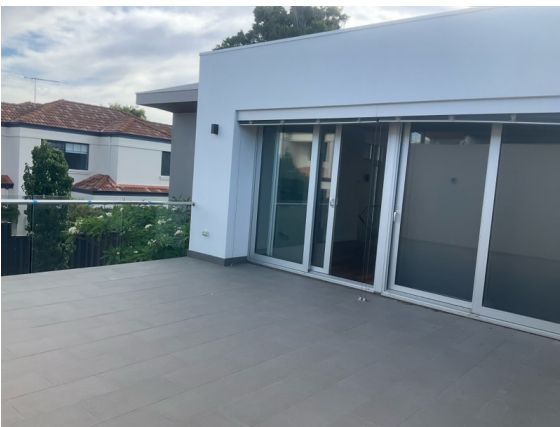
Balcony and western elevation.
