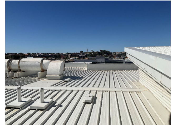
2.01 Roof sheets were assessed to be in good condition
