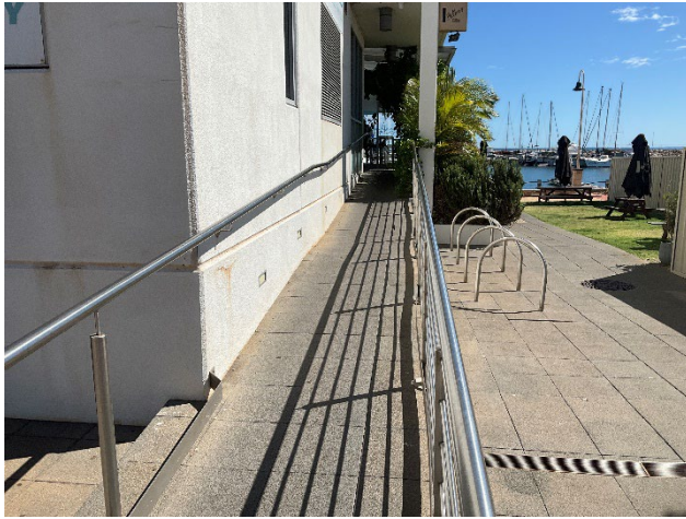
5.01 Lift and reset dislodged pavers to commercial tenancy area.
