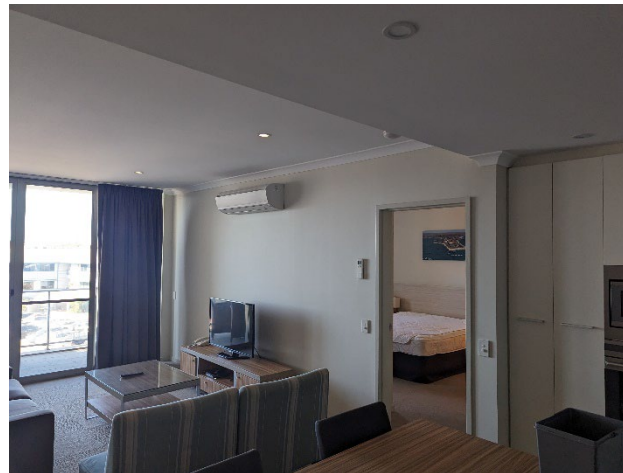
6.02 Apartment wall split
