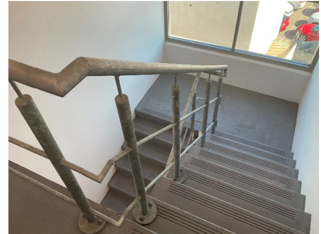
4.20 2No Internal Stairwells
