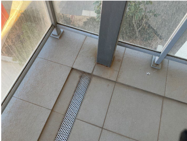
1.02 Painted Steel posts supporting cantilevered balconies
