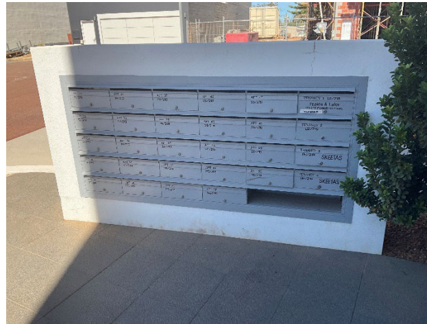
3.12 Masonry structure with 28no lockable mailboxes
