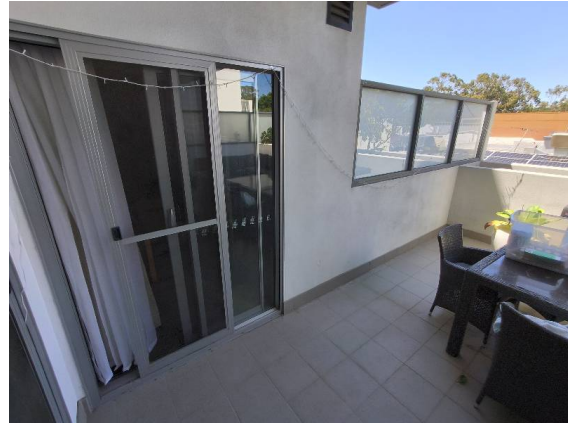
Fiore Apartments - Unit 5 Balcony: View of sliding door to Bed 1.
