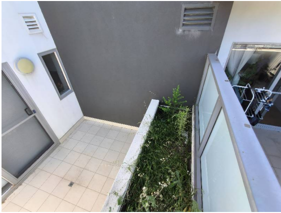
Fiore Apartments – Unit 5 Balcony: Adjoining balcony directly behind Bed 2 of Unit 5.
