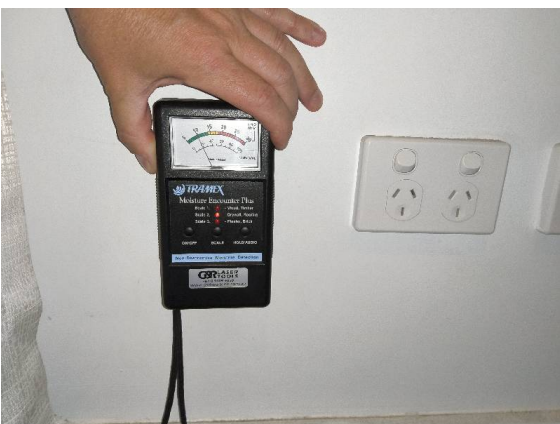
Fiore Apartments - Bedroom #1: Control moisture reading taken at 10%.
