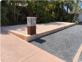
Item: Retaining walls
