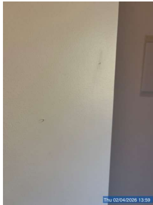
ENTRY: Walls (photo 1 of 3)
