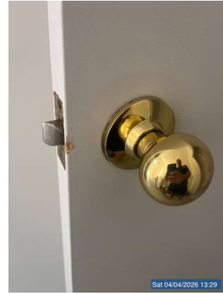
LAUNDRY: Internal Door (photo 1 of 1)
