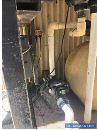
REAR: Pool house/equipment (photo 1 of 1)
